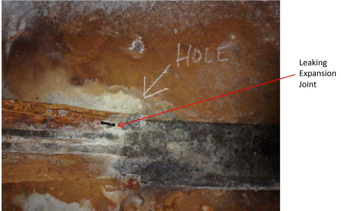
Figure 3: Boiler Ductwork Expansion Joint
