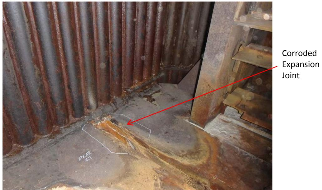
Figure 14: Boiler Ductwork Expansion Joint (2)
